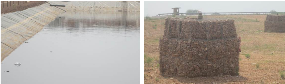
Fig 9.2. Anaerobic pond for leachate treatment & gas extracting structure at Kpone dumpsite
